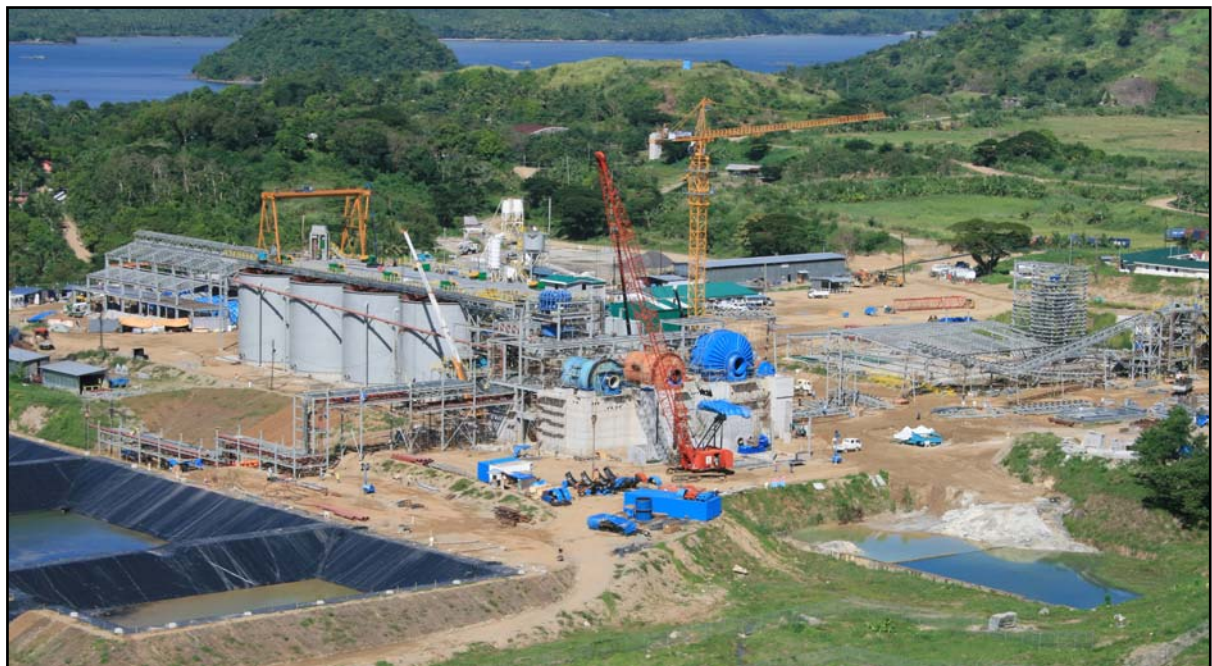
Masbate Gold Project Plant Site
